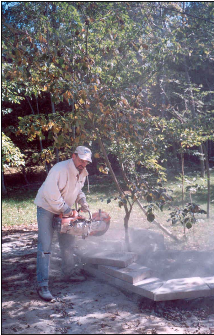
More stone work! Above: Mark used Bradfield's saw to cut cap-stones to shape. Top right: An October view of the completed front wall after the raised part of the yard was re-seeded. Bottom: The last of the wooden pallets await shipment to the landfill.
